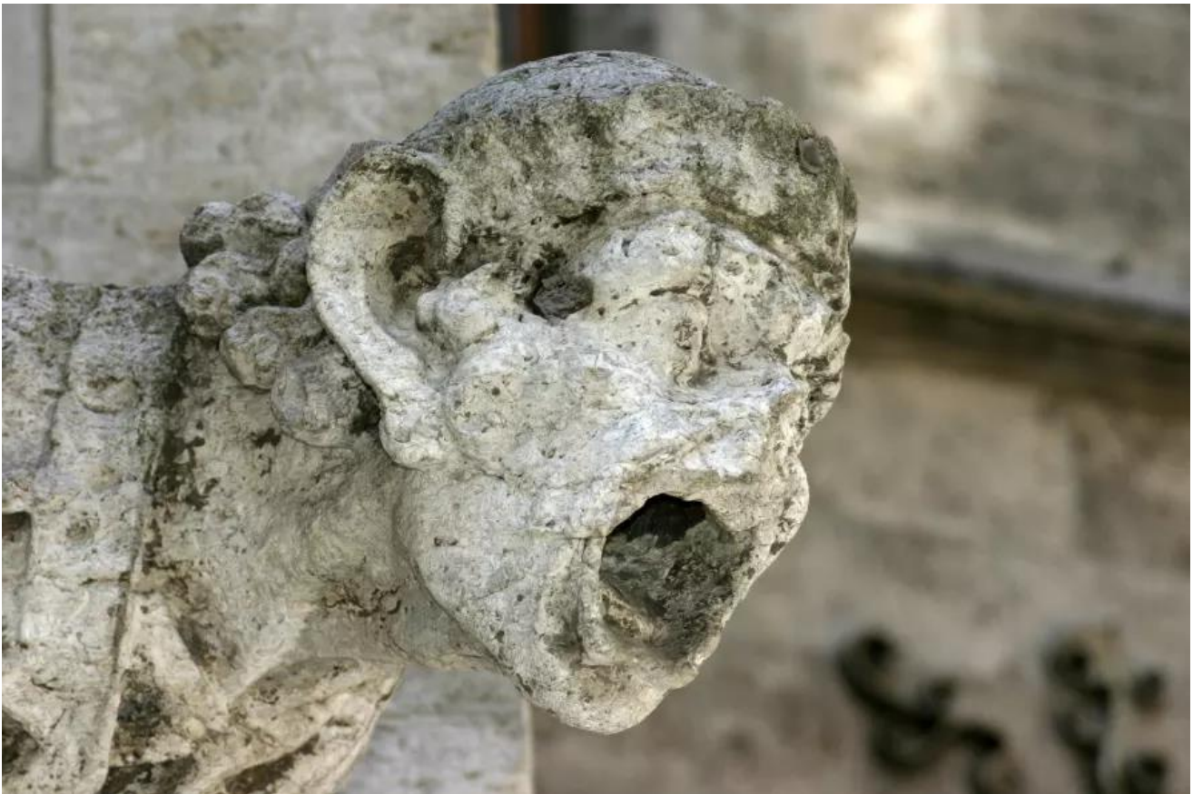
Figure 5.14 A gargoyle damaged by acid rain (Image: Nino Barbieri via Wikimedia Commons)
